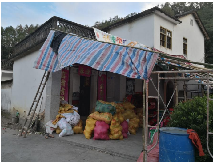
Temporary extension shelter
