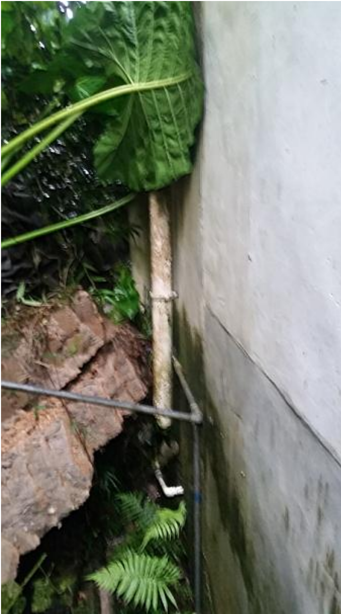
Landslip – collapsed retaining wall
