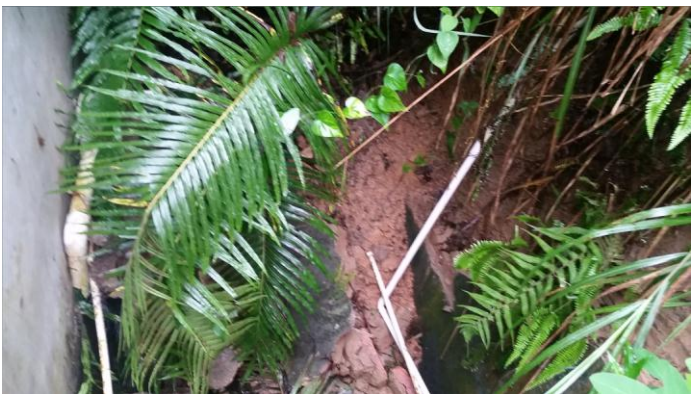
Dislodged water pipes
