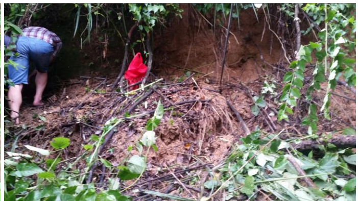
Locating damaged sections
