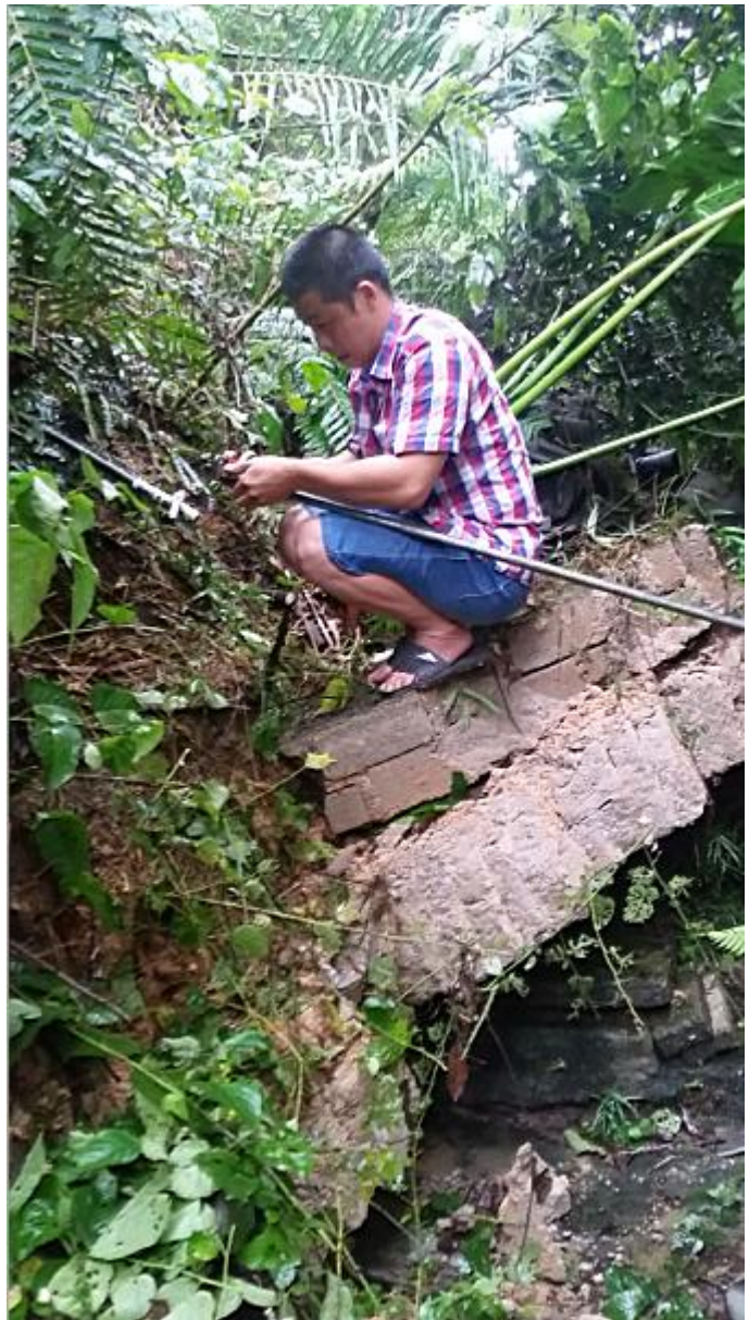
Rejoining broken pipes
